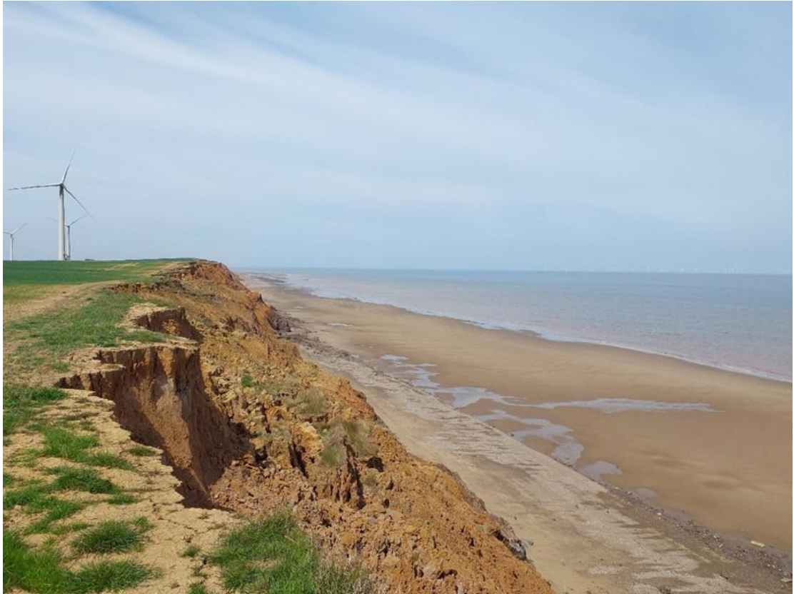
Insert 20-5 – Evidence of Recent Cliff retreat at Easington Landfall
